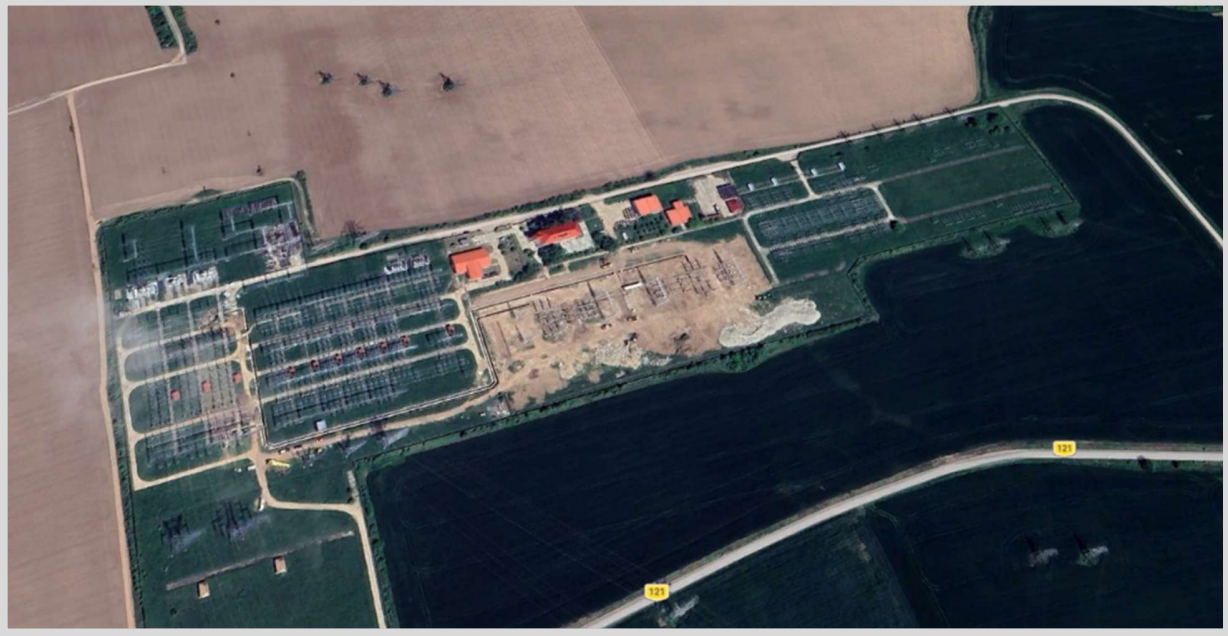
Figure 4-2 400/2200/110 kV Gutinaş Substation
